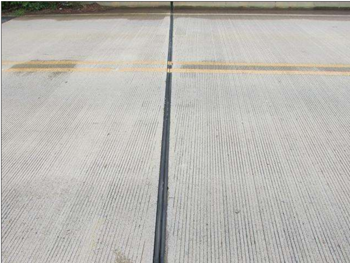
EXPANSION JOINTS AT THE ABUTMENTS AND PIERS
