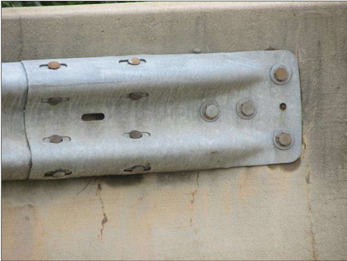
GUARD RAIL CONNECTION SW CORNER ALL SIMILAR
