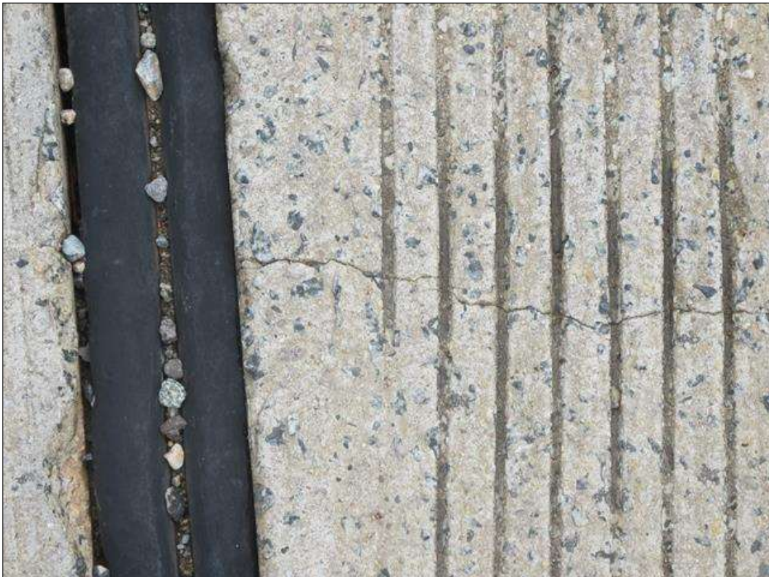
HL. CRACKS IN THE SPAN ENDS
