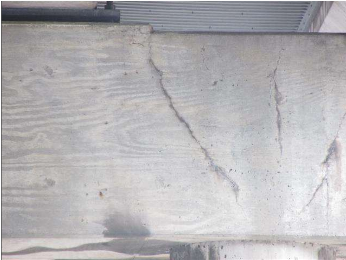
DIAGONAL HL. CRACKS ABOVE COLUMNS 1 AND 2 IN BOTH FACES OF PIER 2 CAP
