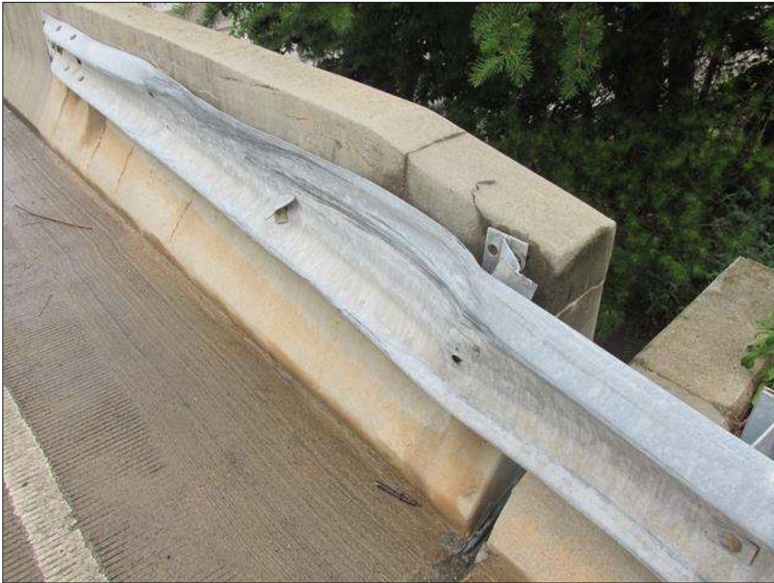
A 20 FT. SECTION OF GUARD RAIL IS DAMAGED AT THE SE CORNER
