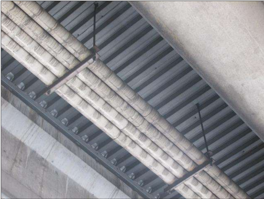
4 - 4" UTILITIES IN BAY 2
