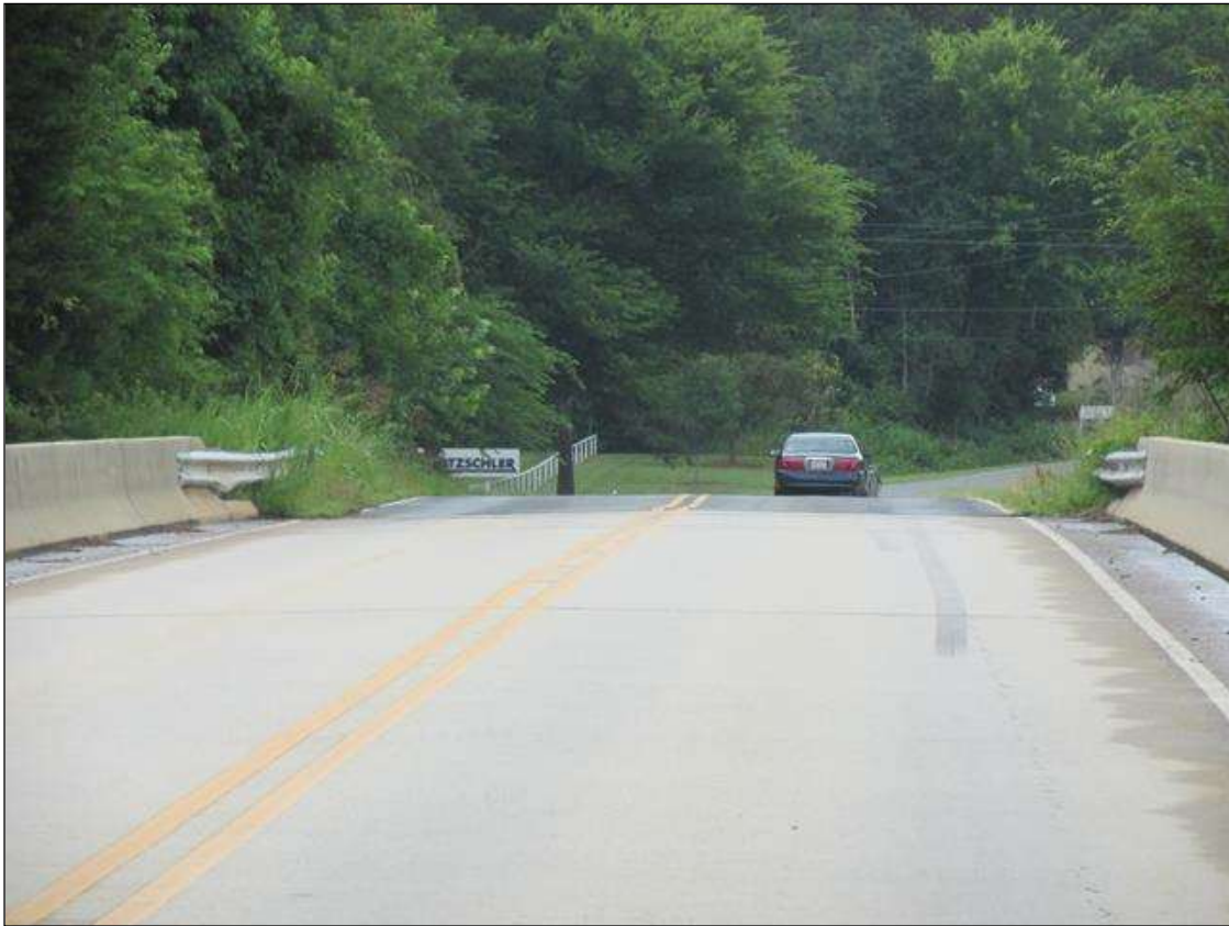
GUARD RAIL LOOKING NORTH
