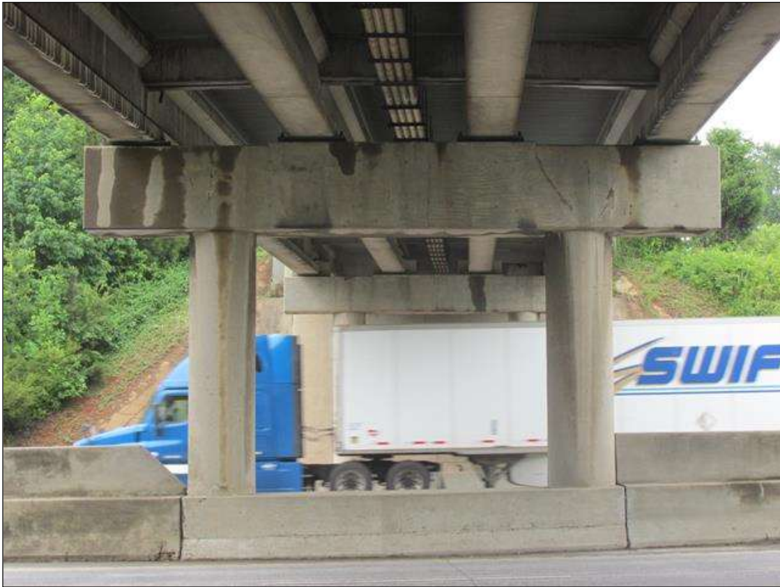
PIER 2 LOOKING NORTH
