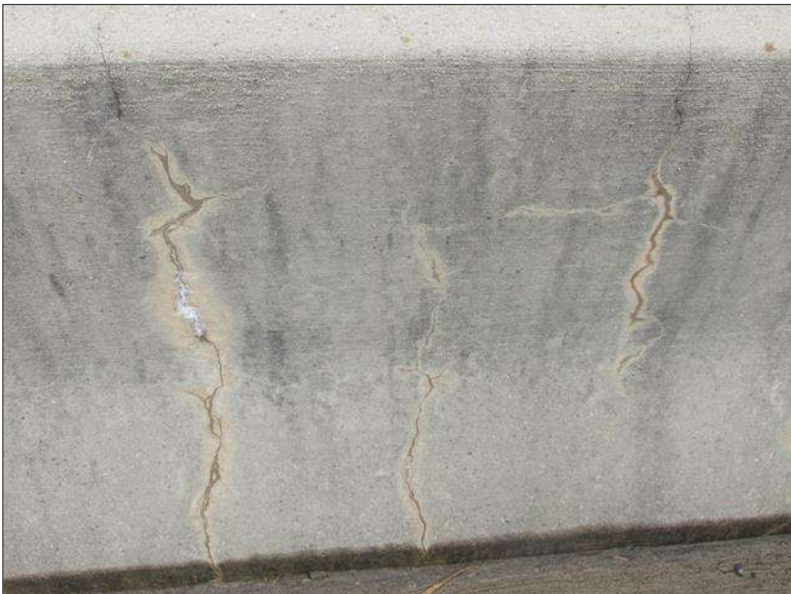
HL. VERTICAL CRACKS IN BOTH RAILS
