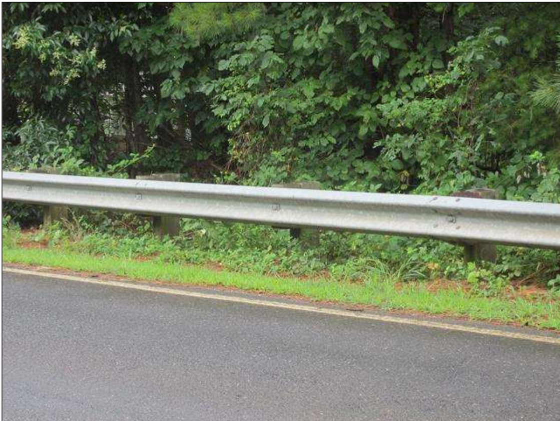
GUARD RAIL POST SPACING IN THE MIDDLE
