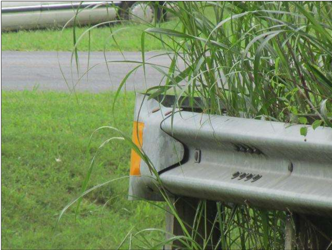
GUARD RAIL TERMINAL END AT THE SW END ALL SIMLAR
