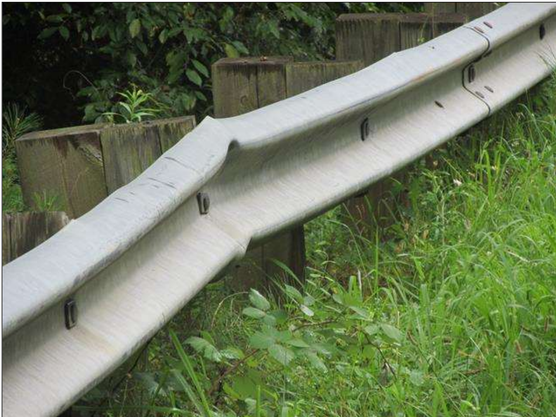
A 30 FT. SECTION OF THE SE GUARD RAIL IS DAMAGED
