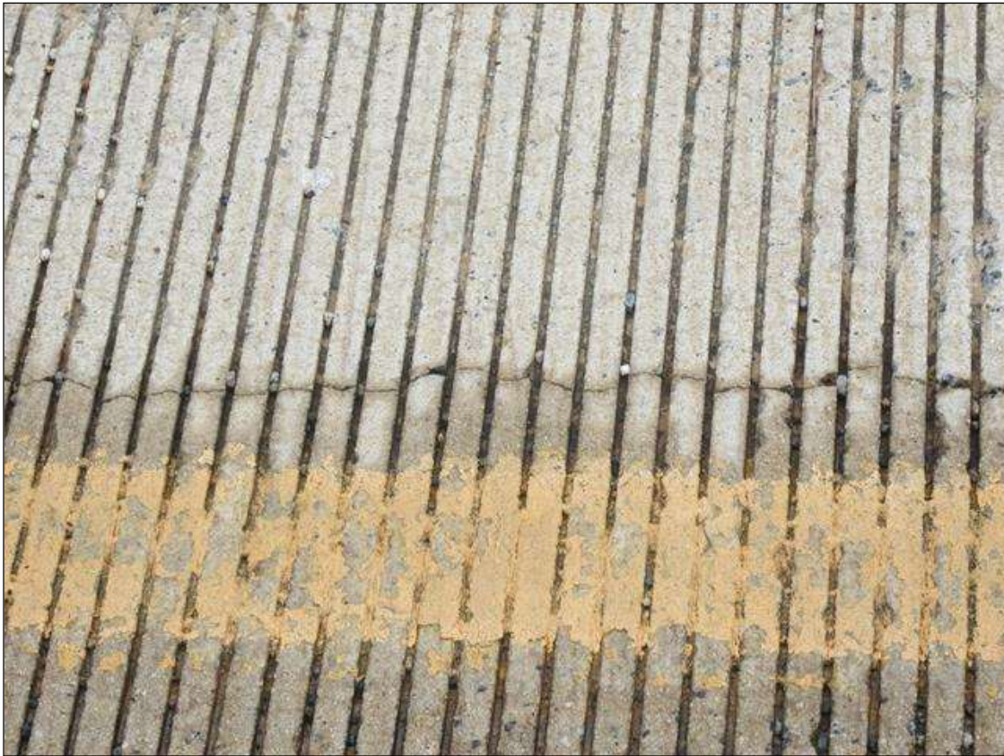
HL. LONGT. CRACKS IN BOTH APPROACH SLABS
