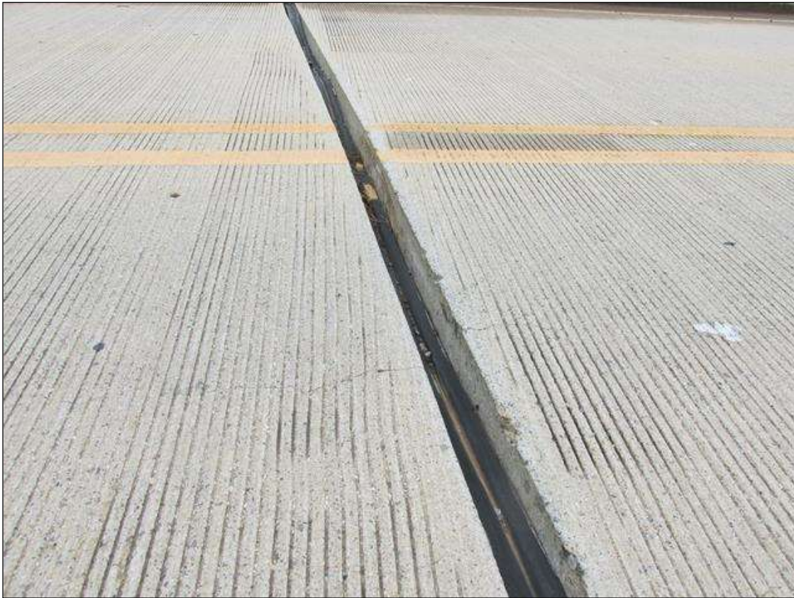
THE EXPANSION JOINT AT PIER 1 IS SETTLED UP TO 6" AND LEAKING
