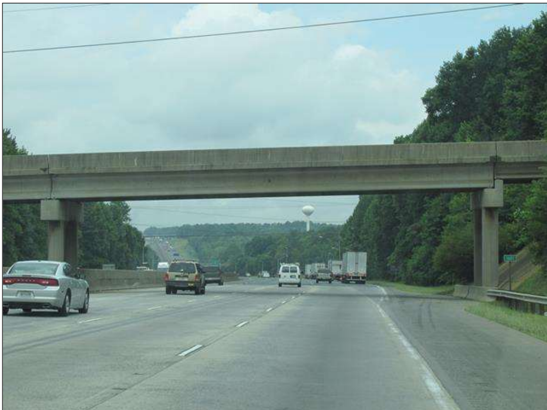
WEST OPENING, SPAN 3
